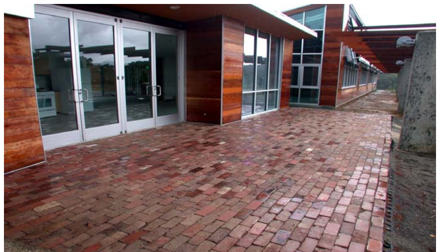
WALKWAY MADE OF 120-YEAR-OLD SALVAGED BRICKS AT THE LESLIE SHAO-MING SUN FIELD STATION. Courtesy of Jasper Ridge Biological Preserve
